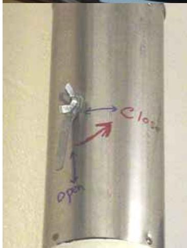
2. Make sure the vent is turned on by turning the lever so that it points down (see picture).
